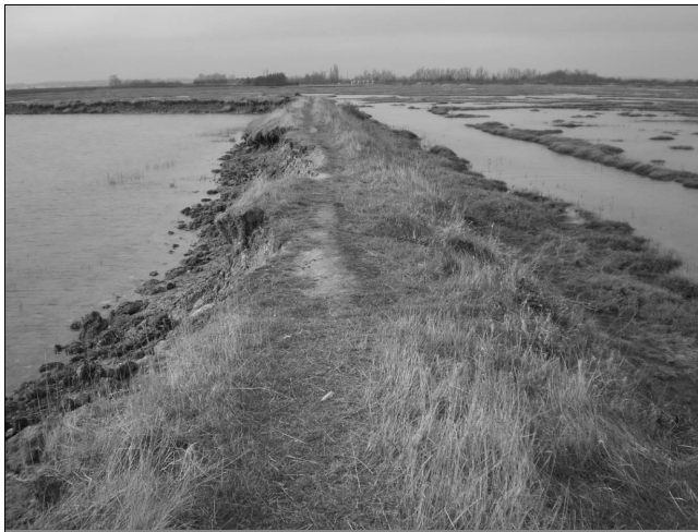
Fig. 3. A former sea wall at Tollesbury. The eroding side is within the realignment site and illustrates the impact of internal wind-driven waves. On its outer face there is no erosion because of the energy absorption of adjacent saltmarsh
